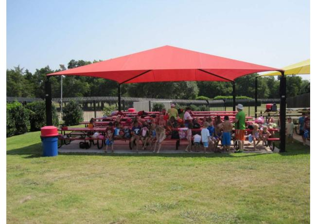
NOTE: PROVIDE A MINIMUM OF 10'-0" CLEARANCE UNDER THE LOWEST PORTION OF THE SHADE STRUCTURE -THE ACTUAL HEIGHT OF THE SHADE STRUCTURE TO BE COORDINATED WITH THE OWNER'S PLAYGROUND VENDOR TO ENSURE MINIMUM CLEARANCES ARE HELD.
